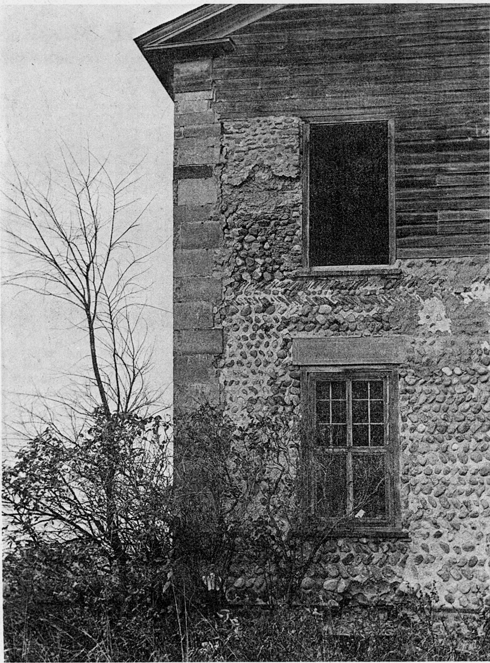
Side wall in various stages of deterioration: Wood siding has replaced some of the lost stones. Note the different sizes of cobblestone under the first-floor window, and herringbone pattern under the second-floor window.
